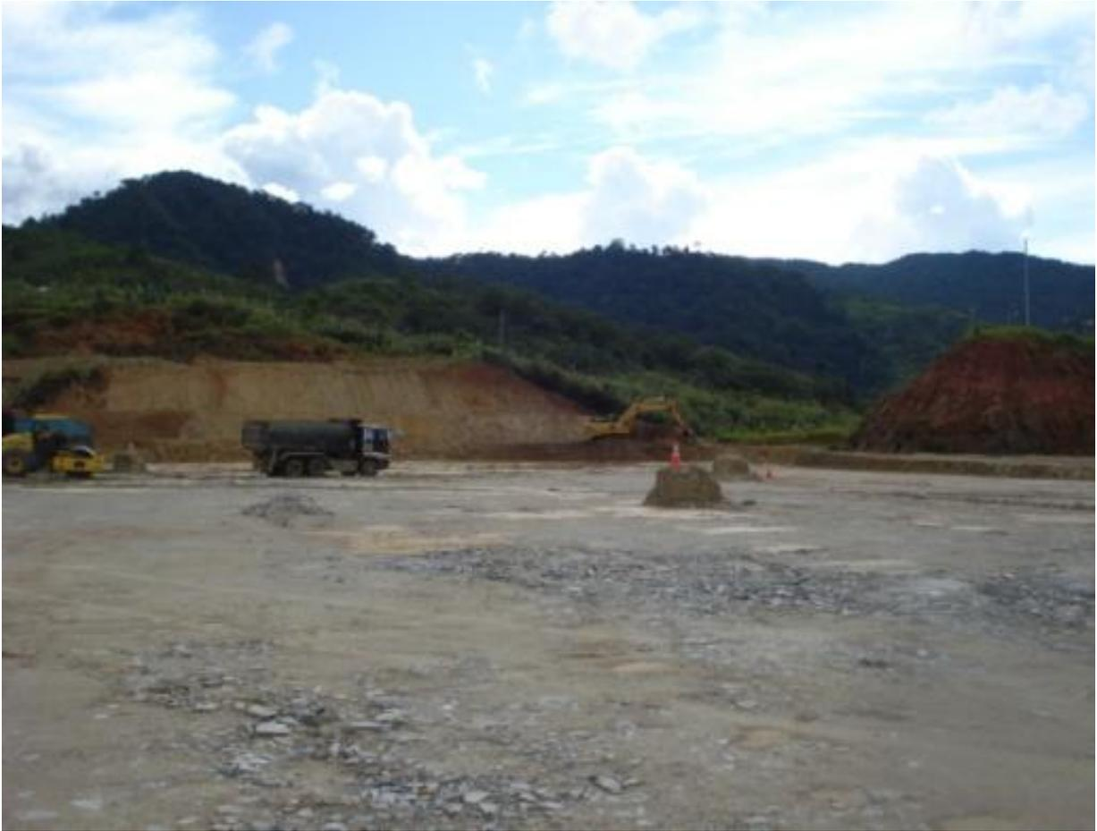
**Figure 3 – Process Plant site preparation and compaction**
