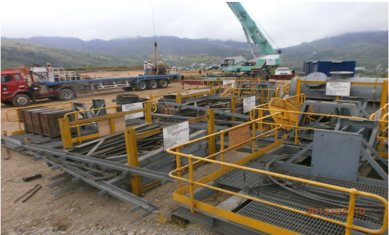
Figure 5 – Process Plant equipment being unloaded at site
