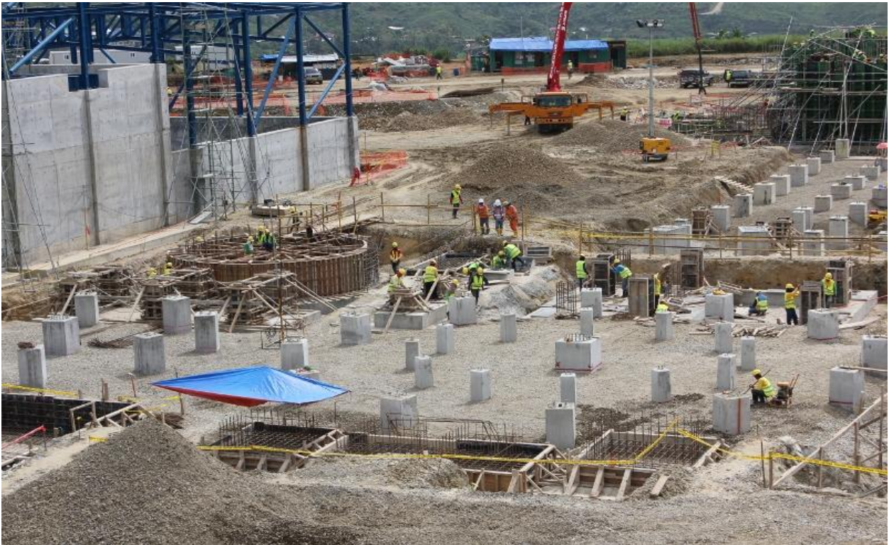
Figure 4 – Footings well advanced for flotation circuit and tank base.
