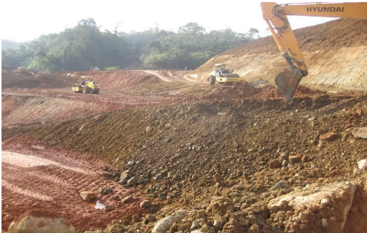
Figure 6 – Construction of TSF embankment
