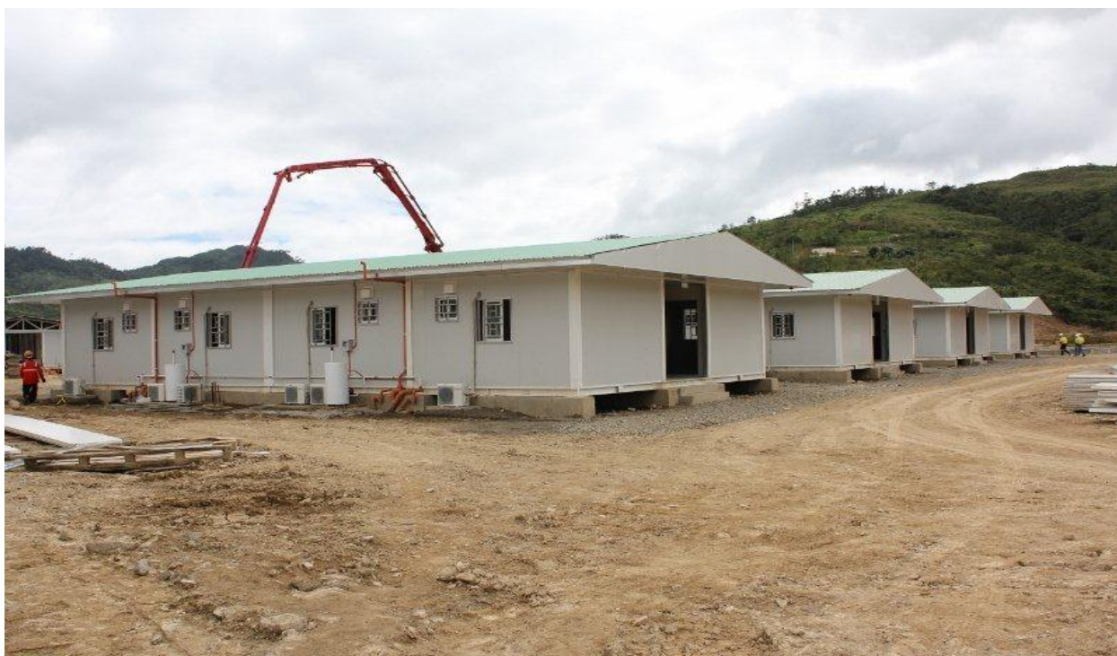
Figure 7 – Staff accomodation for 500 workers completed
