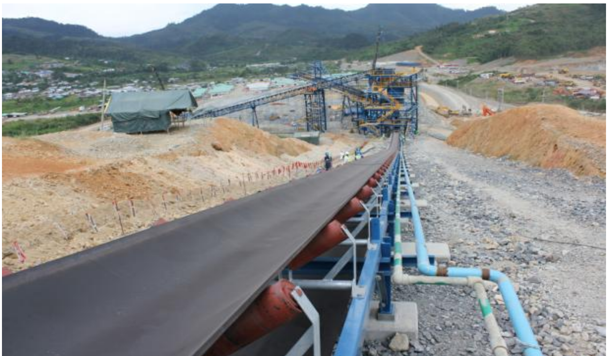
Figure 3 – Conveyor Belts Installation Underway
