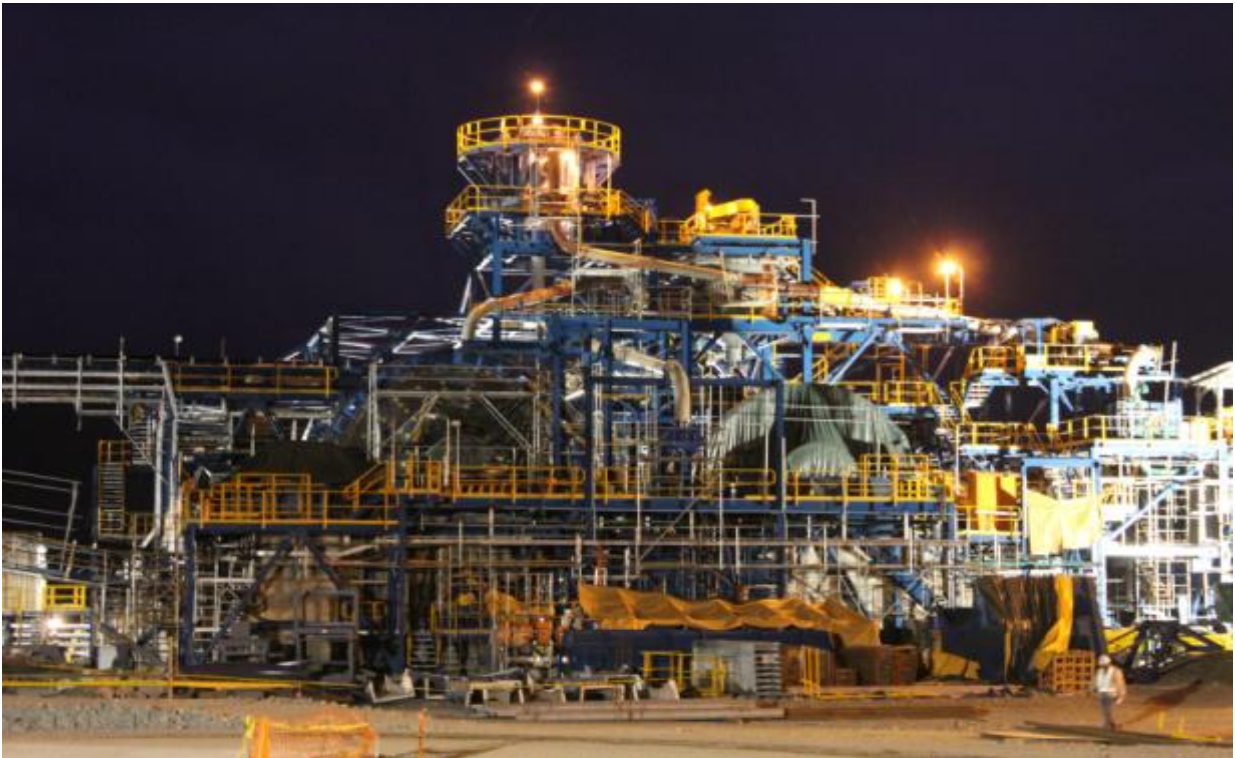
Figure 4 – Grinding Area of Process Plant
