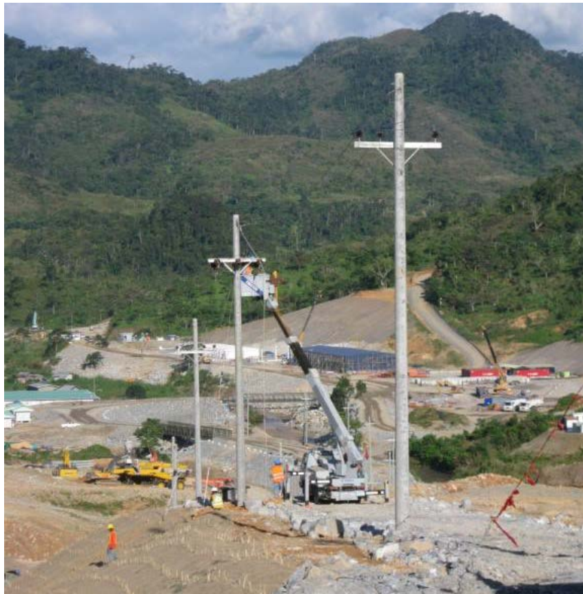
Figure 2 – Power Lines Being Installed to TSF
