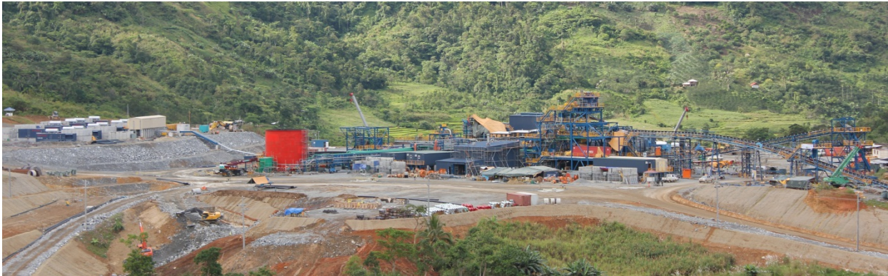
Figure 1 – Plant Site Overview (Oct 1)
