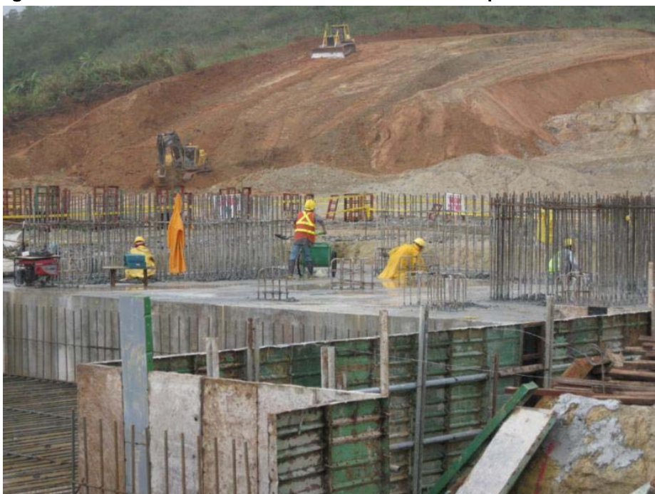
Figure 2: Ball mill foundation with bulk earthworks for power station in background
